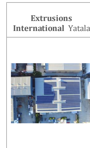
172kW Solar System
